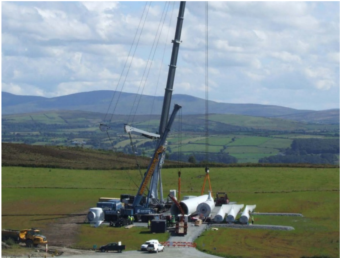
Plate 4.4: Wind Turbine Erection 2
