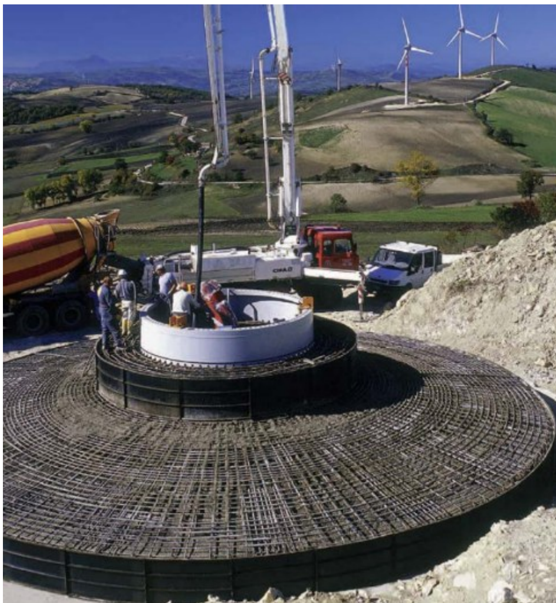
Plate 4.3: Wind Turbine Foundation
