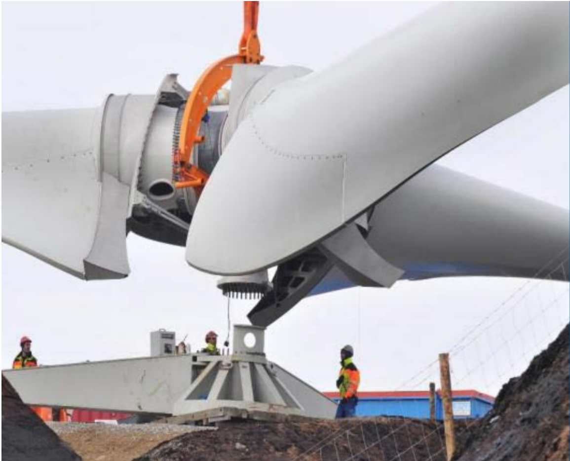
Plate 4.5: Assembly of wind turbine blades 2
